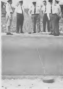
THIN, GRAY strips of hoses are stretched across the road. A car passing over the hoses activates and stops the electric impulse that registers travel time between the hoses.
